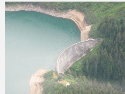
Salmon Creek reservoir and dam. Photograph by Nwchar.
